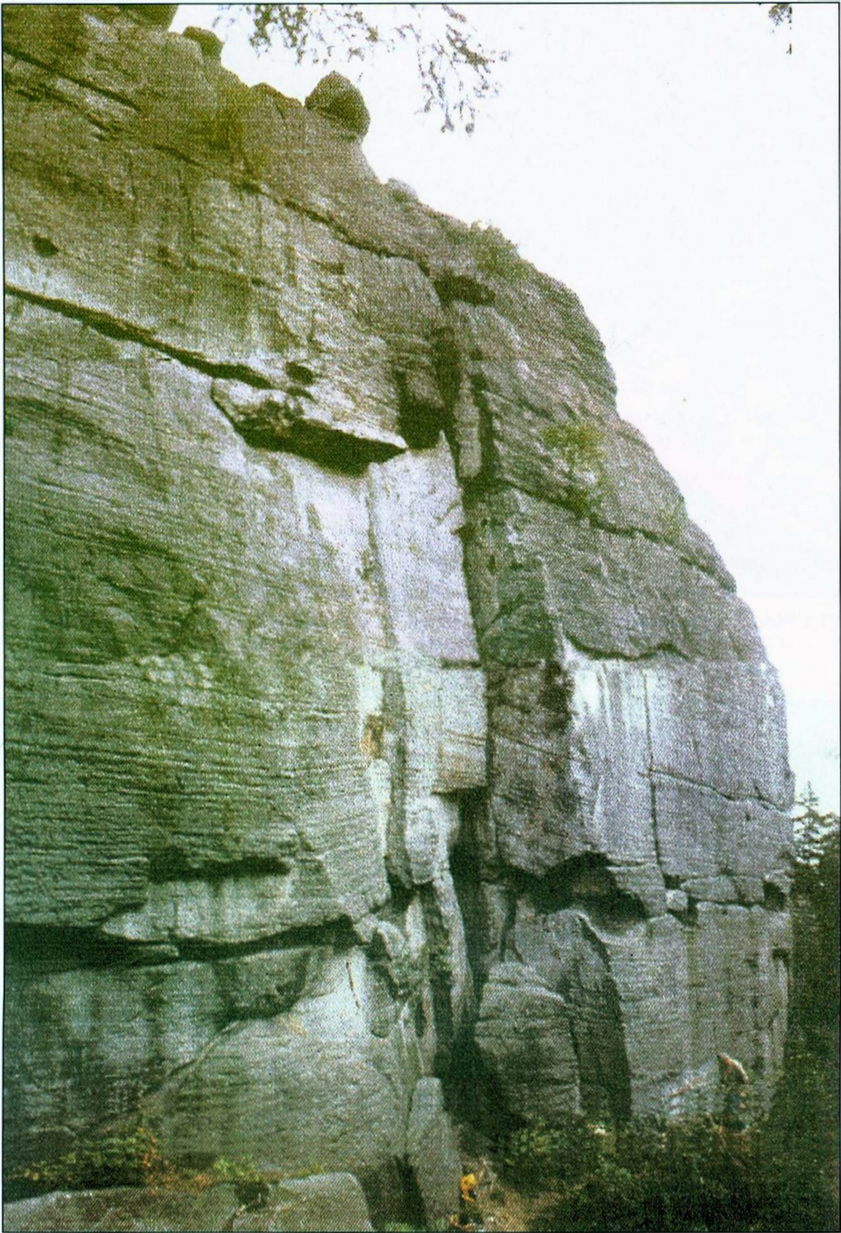
Phot. 2. Marginal rock wall on SE of Szezeliniec Wielki massif showing morphological signs of rockfalling. Crack gauge TM71 installed at the toe. (phot. B. Košťák)
