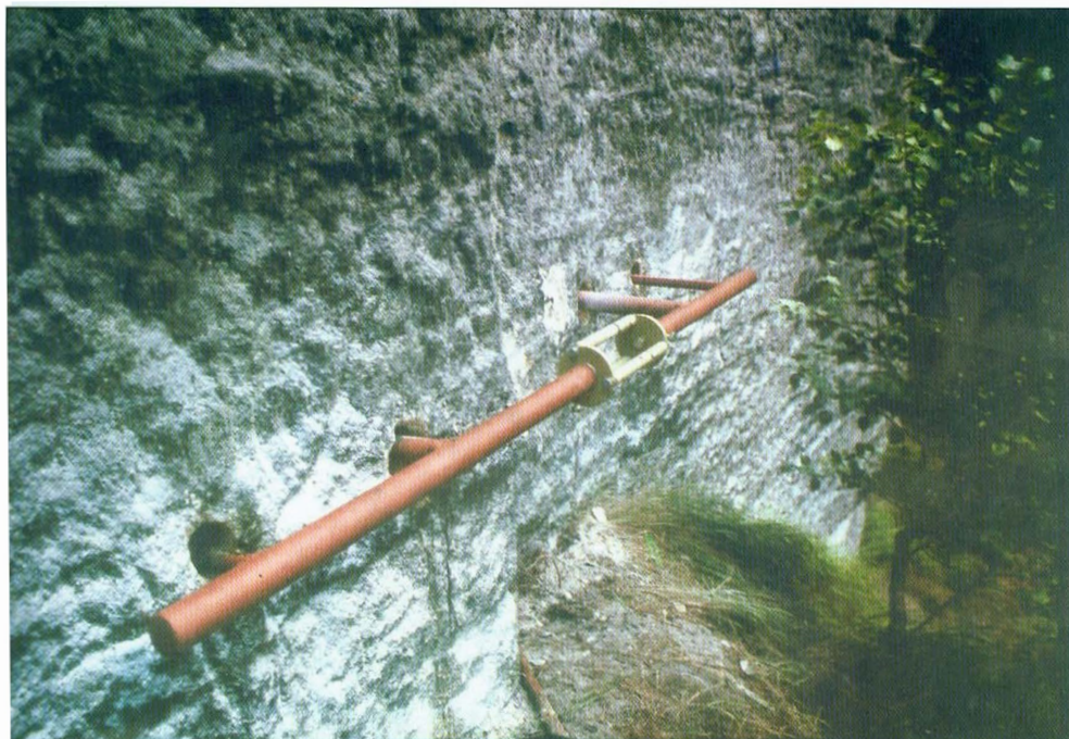
Phot. 1. Mounting the crack gauge TM71 on the crack in the rock wall of locality Schody - Stary Szlak (phot. B. Košťák)
